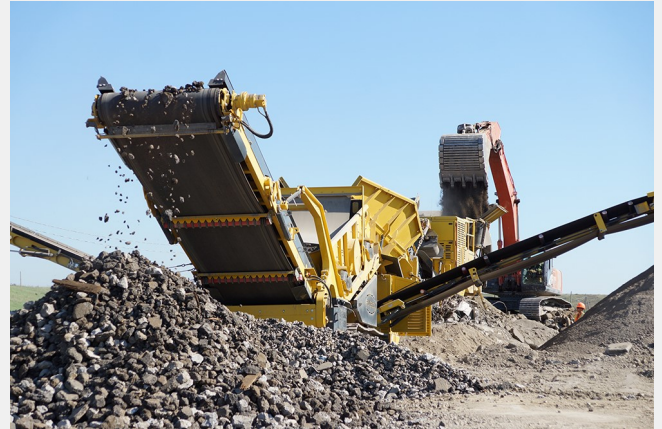
On site concrete recycling
